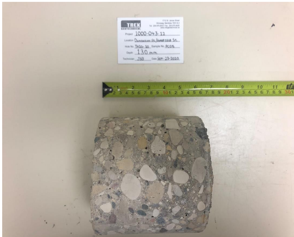
Photo 2: Pavement Core Sample at Test Hole TH20-10
