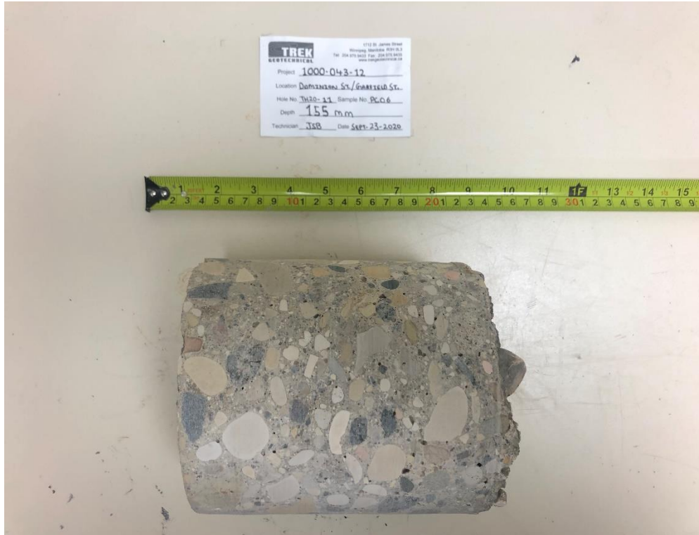
Photo 3: Pavement Core Sample at Test Hole TH20-11
