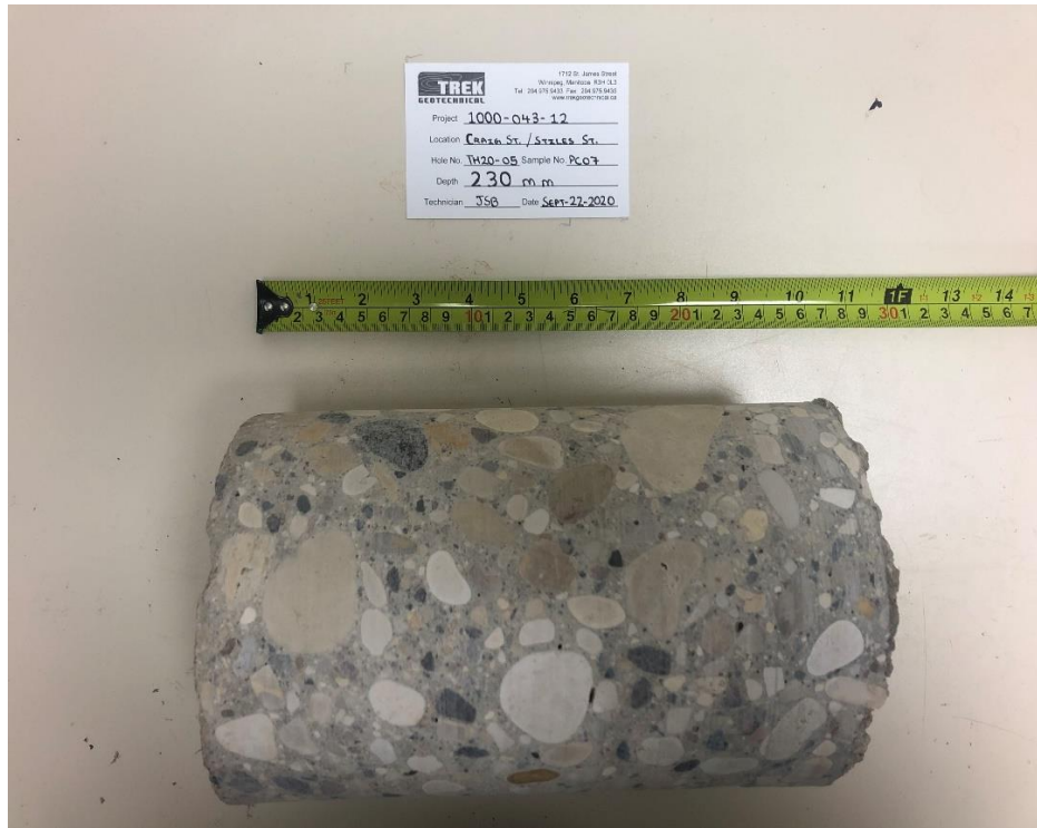
Photo 1: Pavement Core Sample at Test Hole TH20-05
