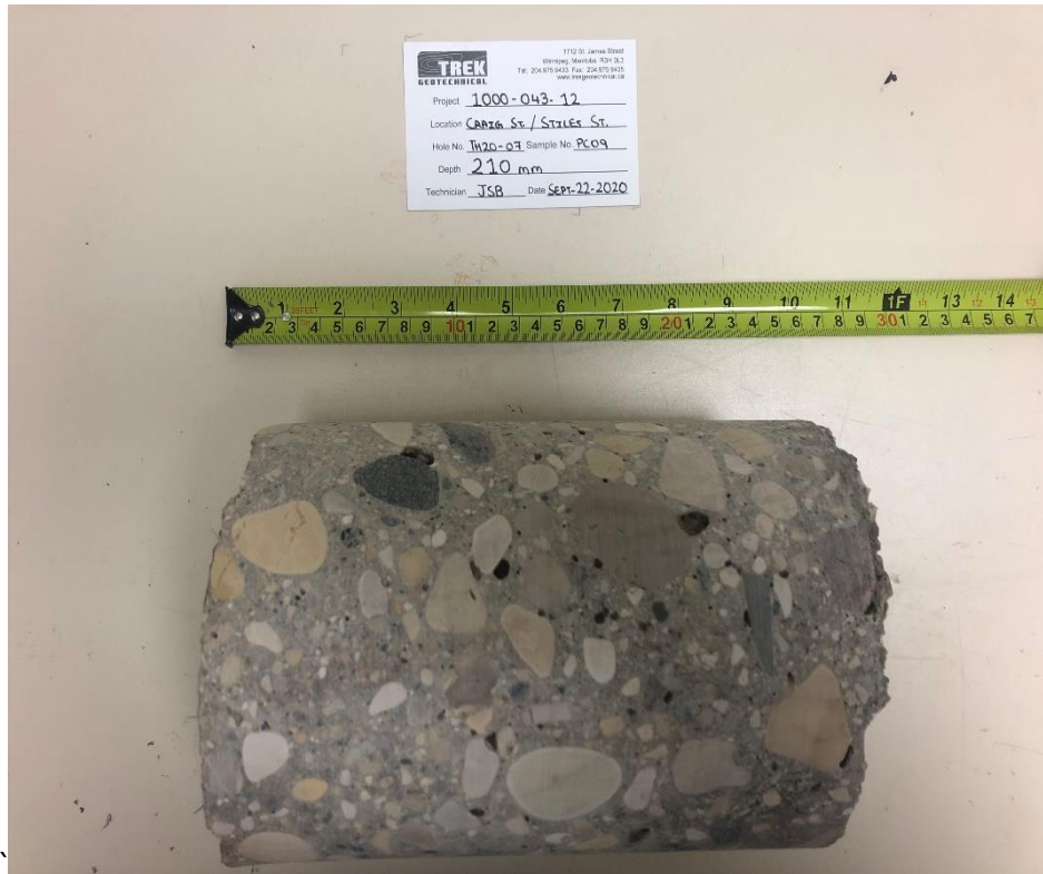
Photo 3: Pavement Core Sample at Test Hole TH20-07
