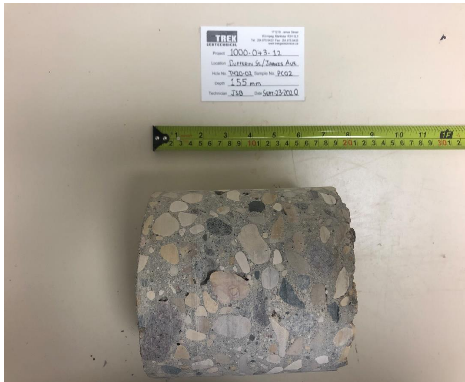
Photo 2: Pavement Core Sample at Test Hole TH20-02
