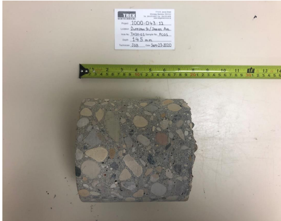
Photo 1: Pavement Core Sample at Test Hole TH20-01
