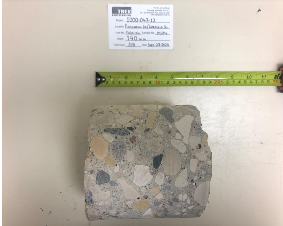
Photo 1: Pavement Core Sample at Test Hole TH20-04
